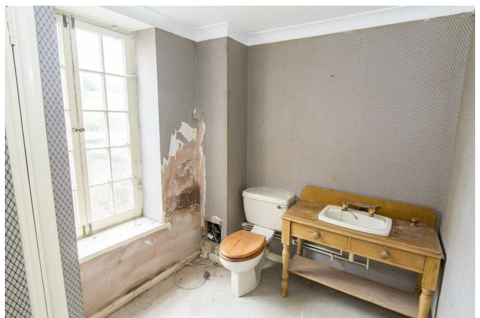
Ground Floor Bathroom 9'8 x 6'10 (2.95m x 2.08m)
